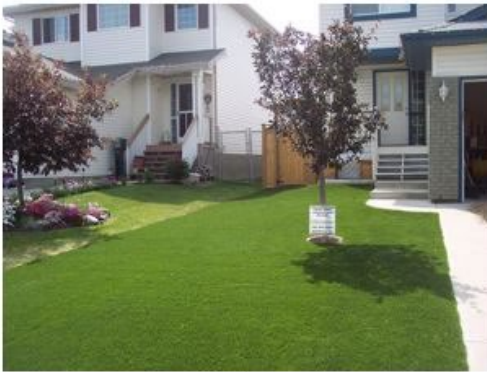
Incorrect – There should be a distinct boarder installed between the artificial turf and the neighboring natural sod.
